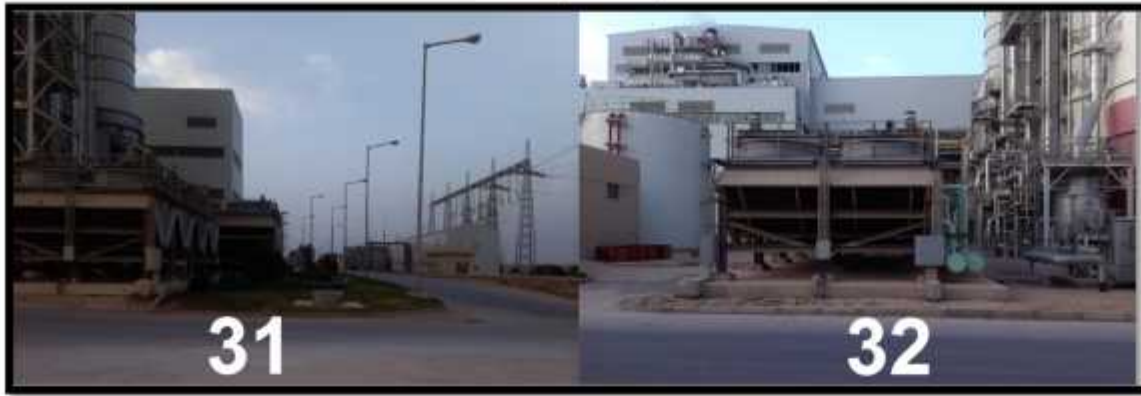
Figure9 place of generator cooling system for GT31 and GT32
